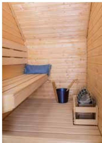
sauna tucks under a stairway, with full-platform middle bench, custom sloped ceiling, and a Junior or Piccolo heater through the lower bench.
