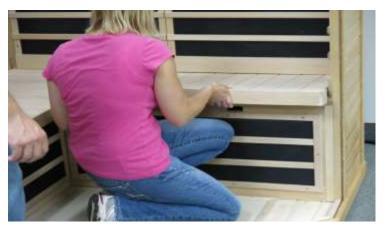
• The Bench Top should fit down flush from front to back. It may be necessary to use the openings in the skirt to apply pressure forward or rearward on the skirt to allow the bench to drop into place.
