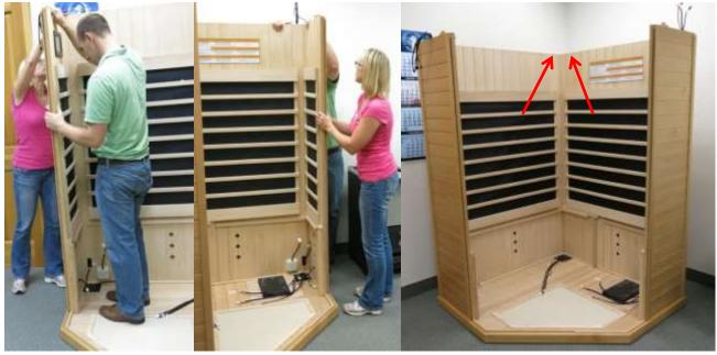
Note: When wall panels are connected in place properly the corners will be level and flush on top.
