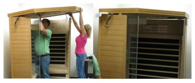
• Once the Ceiling panel is lined up directly above the Wall panels; insert the wires harnesses from the wall panels into the holes in the Ceiling panel.
