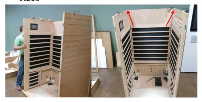
Note: When wall panels are connected in place properly the corners will be flat on top, notice the illustration above right. The right wall is incorrect; the left wall is the correct installation.
