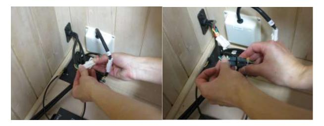
• Connect wire R1 from the distribution plate to R1 from the Right Wall junction box.
